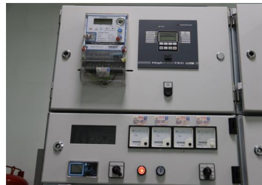
Microprocessor relays and smart meters
